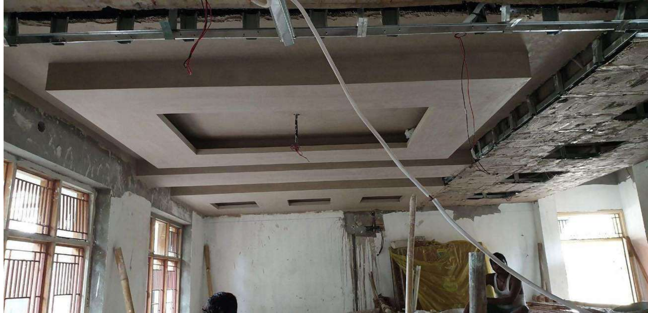
Execution Home Office (False Ceiling)
